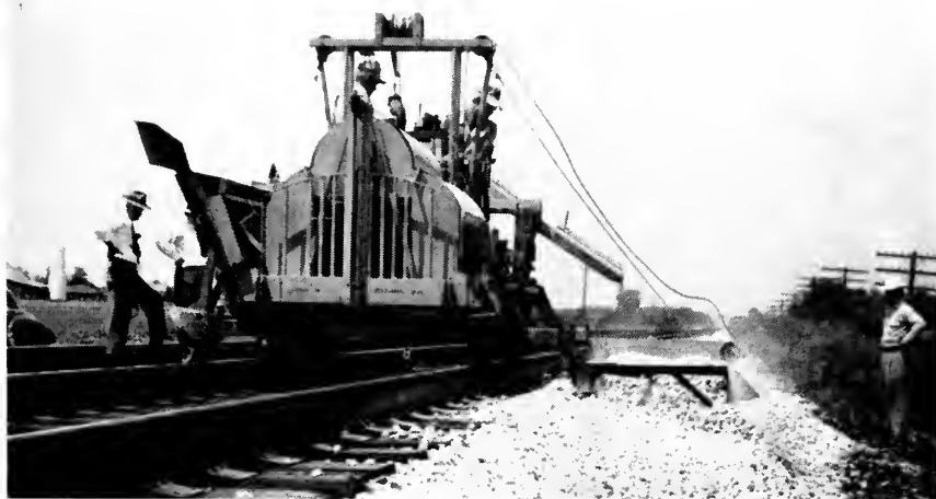
Another view of machine for regulating and plowing ballast.
